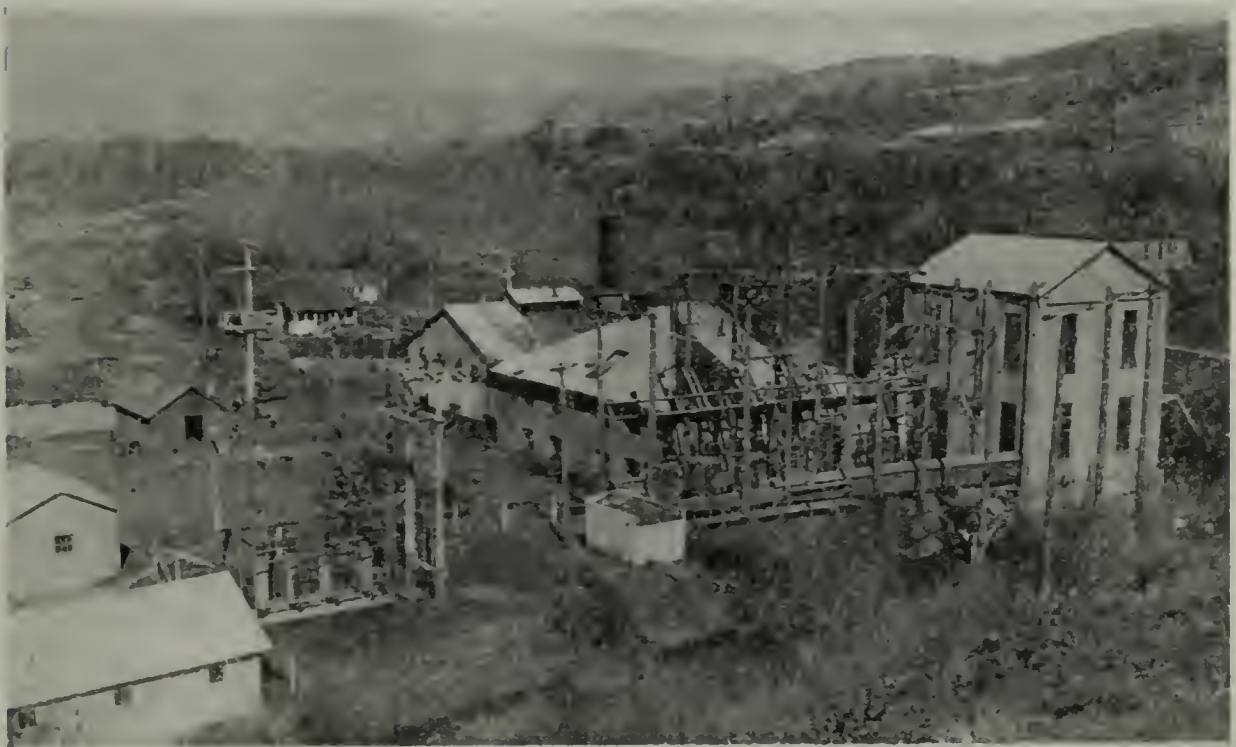
Naches Generating Station - December 31, 1936
